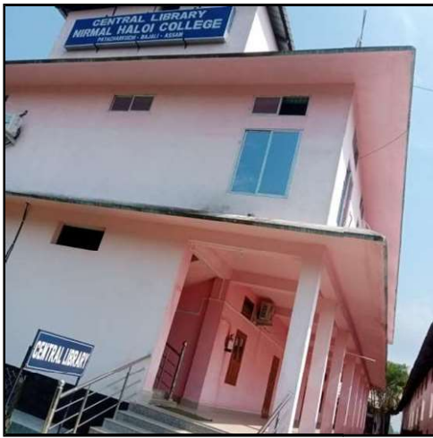
Library Outside View
