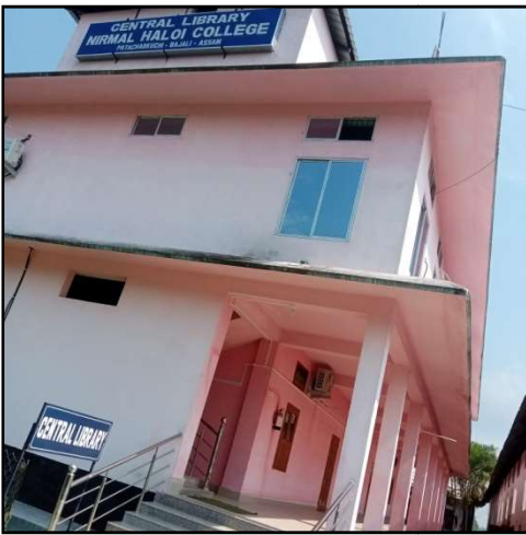
Library Outside View
